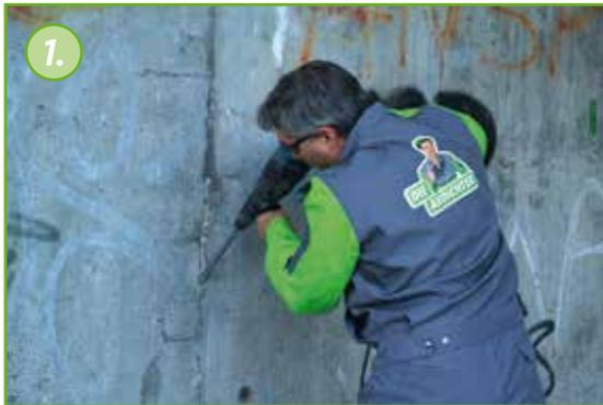
Open the crack in a V-shape 1 cm to 2 cm deep and remove loose particles and dust with a brush.
