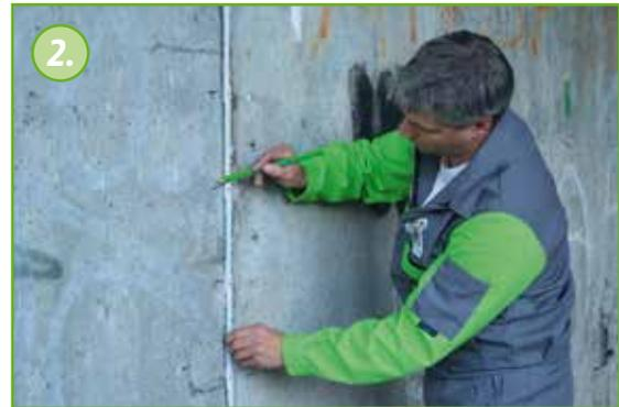
Mark the positions where the boreholes are going to be drilled. Boreholes are placed along the course of the crack on alternating sides at intervals of approx. 10 cm to 15 cm.
