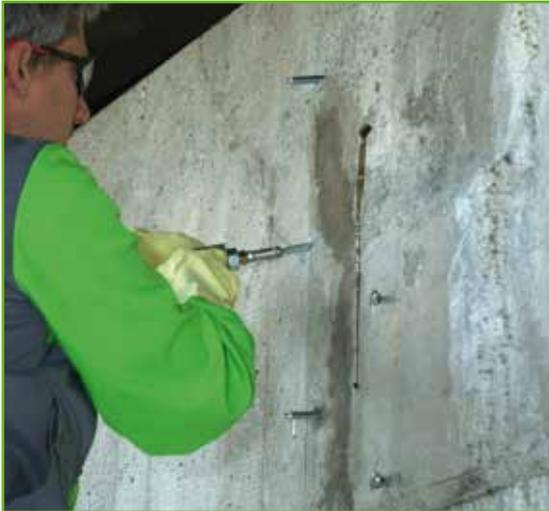
1. Prior to the injection, every third borehole is left open. When KÖSTER 2 IN 1 is injected via an injection packer, it can travel through the crack to the open borehole next to that injection packer. Enough material has been injected into that particular injection packer, when KÖSTER 2 IN 1 comes out of the next open borehole.
