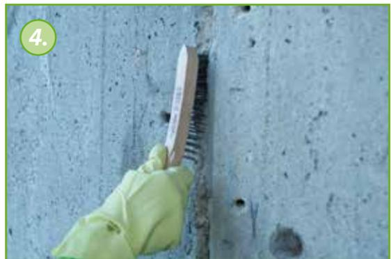
Clean the crack using a wire brush.
